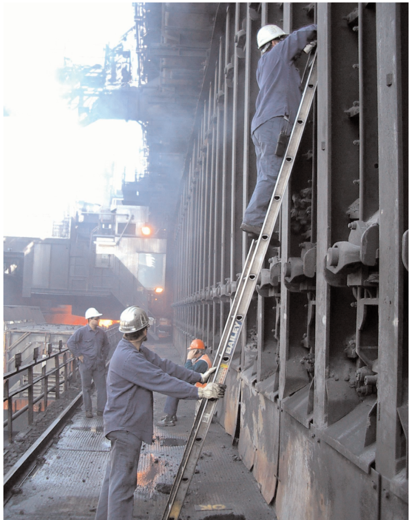
Photograph 1. Specialists adjusting battery doors
